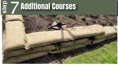
Repeat steps 3-6 until you reach your desired bed height. Be sure to set the bags in a brick pattern, so that the bag above spans the seam between two bags below by at least 8". Backfill behind each course once completed. Level each bag as needed by adjusting the snorkel wrap length.
