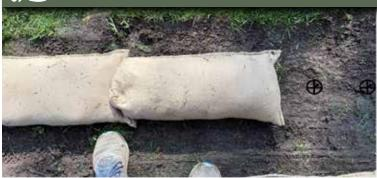
Place the pins along the trench, spacing them 12-18" apart. Next, place the first course of bags over the pins, so two pins connect with each bag. It's okay if you need to move pin locations as you go. Be sure the bags fit tightly to one another and the "snorkel" is tucked below the bag.
