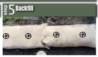
For raised garden beds, a backfill mixture of sand and topsoil work best. Fill the space behind the bags with backfill material and rake level so that the material is 2"-3" higher than the bags. Next, compact the backfill material with a hand tamper until the level is even with the top of the bags.
