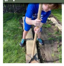
Once the row is in place, use a hand tamper to level and compact the bags. For beds taller than 24" high, we recommend compacting each bag after it is set, as it is easier to level.
